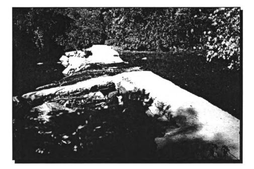
BLOCKAGE NW 6: Sheet-piles, large rock, and gabion baskets topped by a concrete spiliway
