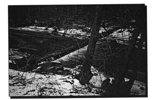
BLOCKAGE RC 8: Active thirty-six (36)-inch, concrete encased, sanitary sewer line
