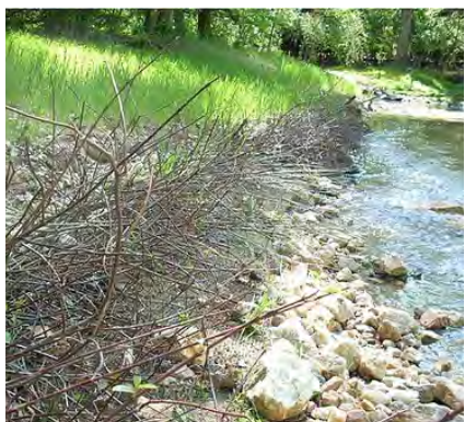
Figure 5-1. Rootwad revetments can be effective in protecting the toe of the slope, as well as providing fish habitat, and collecting sediment and debris (source: Montgomery County, MD "Stream Restoration Techniques").
