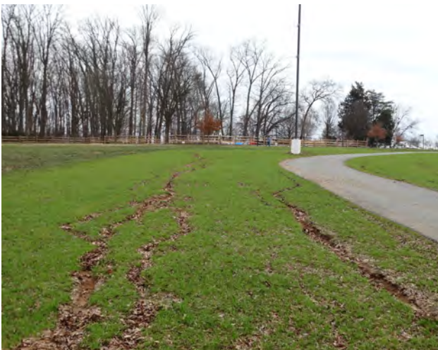
Figure 3-110. Erosion damage on Gil's Hill (QE, 2020).
