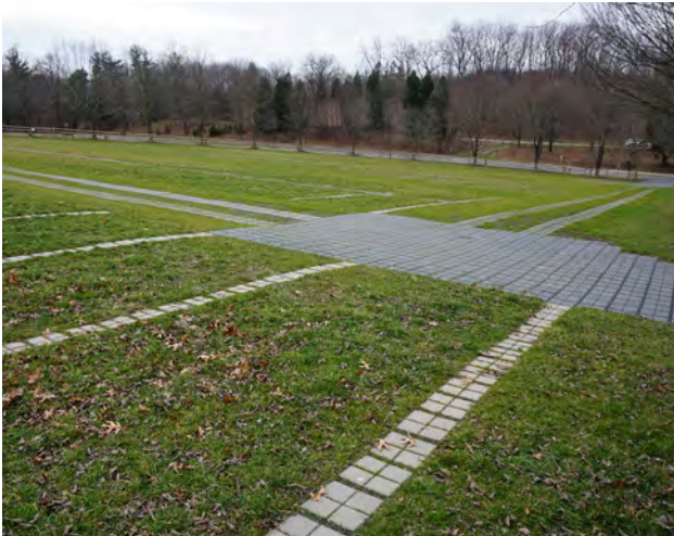
Figure 3-108. Encore Hill grass pavers and parking delineation (QE, 2020).
