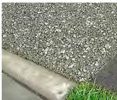
Figure 5-15. Permeable concrete (The Concrete Network).
