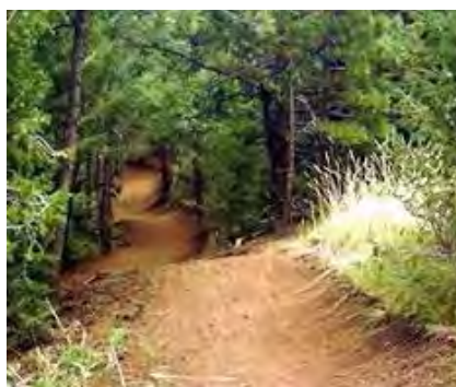
Figure 5-31. Rolling dips implemented on a bare earth trail (San Diego Parks).
