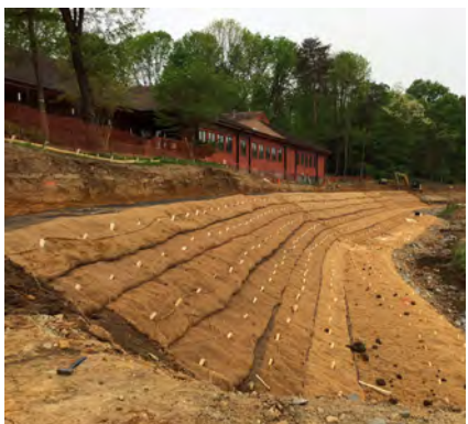
Figure 5-4. Natural fiber matting is appropriate as a temporary stabilization measure as vegetation is established on a bank (source: Hylbrook Park, Prince William County Environmental Services).
