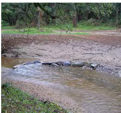
Figure 5-8. J-hook vanes direct erosional forces away from unstable streambanks and improve aquatic habitat by forming scour pools (source: Montgomery County, MD "Stream Restoration Techniques").
