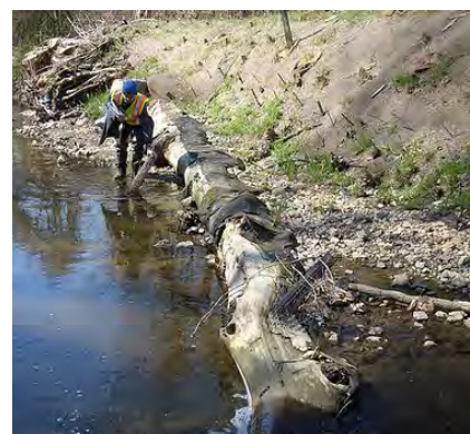
Figure 5-9. Log vanes function similar to rock vanes, but are more appropriate for stream beds with higher proportions of sand, silt, and clay (source: Montgomery County, MD "Stream Restoration Techniques").
