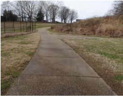
Figure 5-22. 8' wide exposed aggregate concrete walkway, east meadow (QE, 2020).
