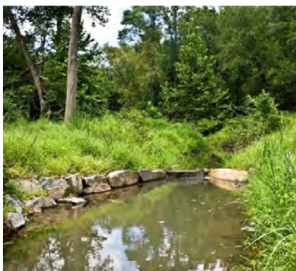
Figure 5-5. Rock revetment structures provide durable protection to the lower portion of the streambank, and may be combined with integrated bank treatment (source: James Long Park, Prince William County Environmental Services).
