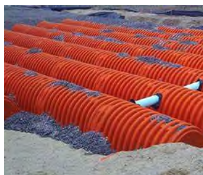
Figure 5-16. Sub-grade retention system (StormChambers).
