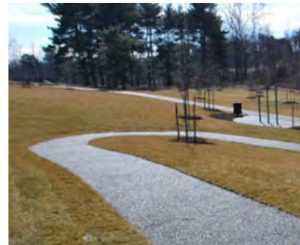
Figure 5-29. Flexi-pave is a heavy duty porous pavement constructed of recycled passenger tires. It can provide an effective low impact and accessible walking surface. Select a color that is compatible with the native soil of the cultural landscape (Capitol Flexi-Pave).
