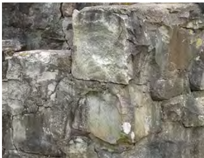
Figure 5-57. Mortared fieldstone, Grill (QE, 2020).
