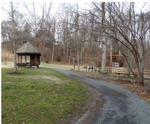
Figure 3-105. Secondary crushed fines over bonded rubber mulch trail within east meadow (QE, 2020).
