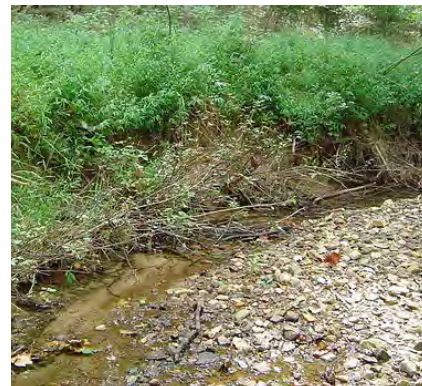
Figure 5-3. Branch layering stabilizes the bank with alternating layers of soil and live branches. Branches extend from the stabilized face of the bank into the original bank material (source: Montgomery County, MD, "Stream Restoration Techniques").
