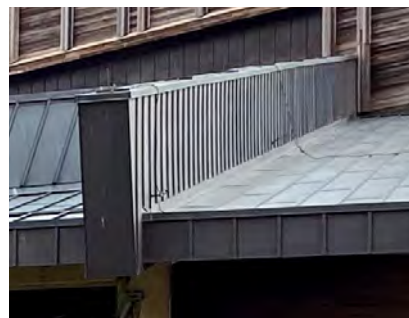
Figure 5-53. Standing metal seam roof, Filene Center (QE, 2020).
