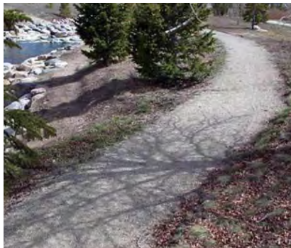
Figure 5-28. Crushed fines of limestone compact over time to provide a safe, accessible surface consistent with the historic character of the site. Surface installation does not require excavation (American Trails).
