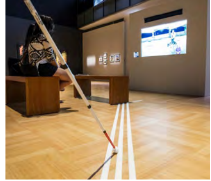
Figure 5-89. Tactile features should support movement through the site. Use changes in texture to indicate changes of direction, wayfinding, and sense of place. Tactile surfaces can also provide access to content through 3D models, reliefs, and braille (QE, 2020).
