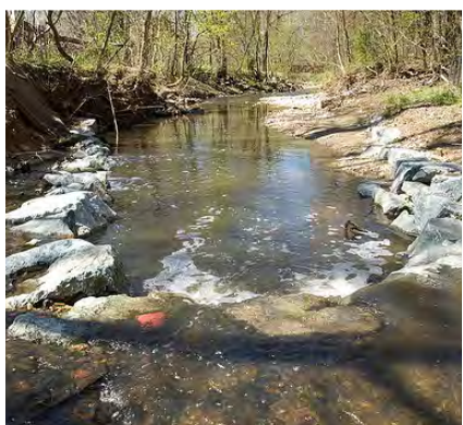
Figure 5-7. Rock cross vanes are constructed to provide grade control and reduce bank erosion (source: Montgomery County, MD "Stream Restoration Techniques").
